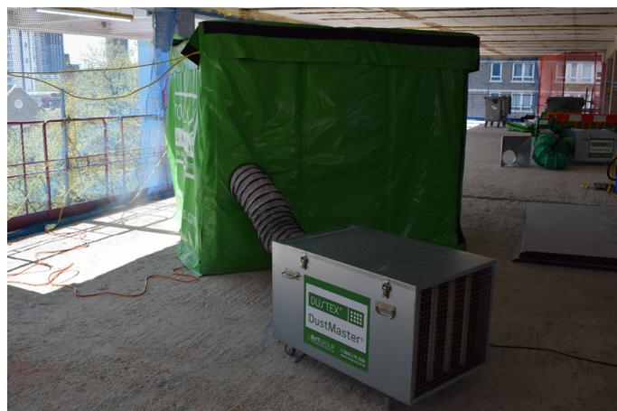
This is another example of a worker using an acoustic enclosure with a dust extraction unit attached to the vent. This ensures that there is minimal dust migration when using the floor scabber.
