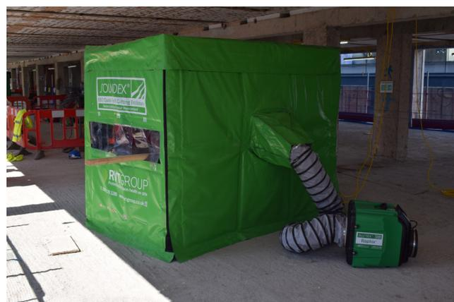
These photos demonstrate how to capture, contain and control dust, whilst also reducing noise on site. The construction worker is using a cutting tool inside a purpose built acoustic cutting enclosure. The cutting enclosure has an aluminium frame with lockable castors and acoustic covers; inside the unit has a cutting bench and an extraction vent. Ducting connects the extraction & filtration unit to the vent, providing an 'all-in-one' dust & noise solution.
