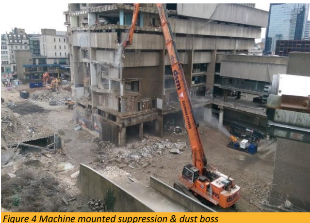
Figure 4 Machine mounted suppression & dust boss
