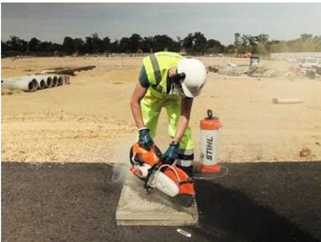
Figure 2: Cutting with controls reduces exposure to dust
