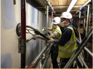
Figure 1: Controls for plasterboard sanding
